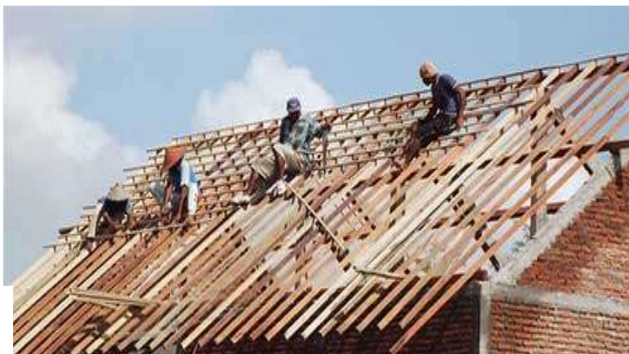
Gambar 3.2 Rangka Atap Kayu (Sumber : Petra Truss April 2016)
