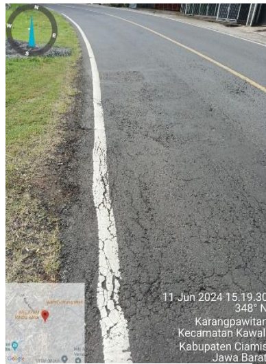
Gambar. (Cracking)
