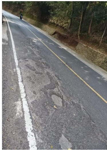
Gambar. (Disintegration)
