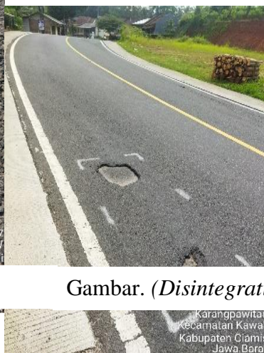
Gambar. ( Disintegration )
