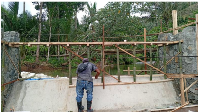
Lampiran 14 Bekisting Jembatan
