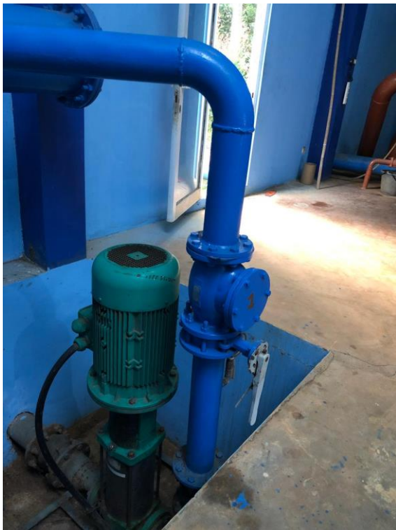
Pompa Sentrifugal Single Stage
